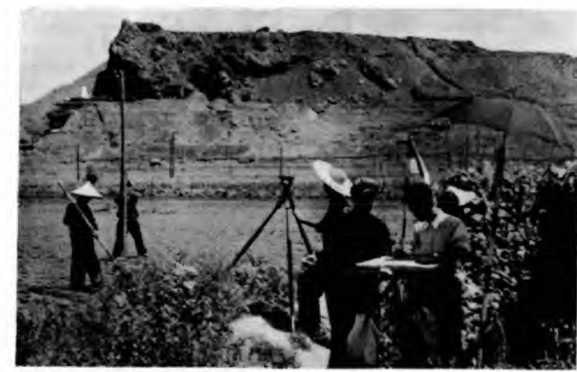
Surveying the fron deposits in Taku Mountain with a view to extending the existing mining area.
